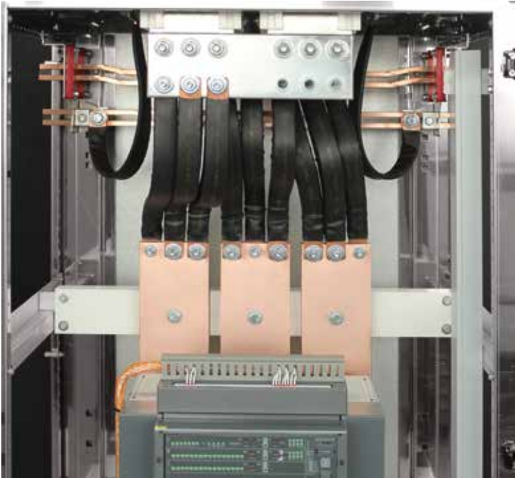
Ultraflexx® for the flexible bridging of bar and power switch
